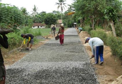
A photograph showing several construction workers on a dirt road. One worker in a yellow vest and black shirt is bending over, using a hand tool to spread gravel. Another worker in a white shirt and blue pants is also working on the gravel. In the background, there are trees, some buildings, and other workers further down the road. |
